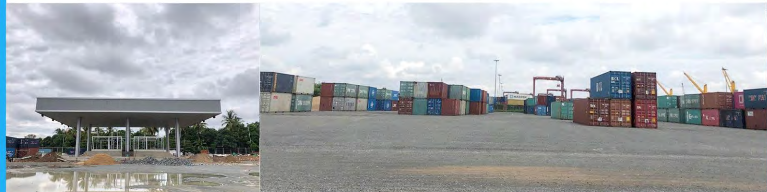
Construction of New Gate
